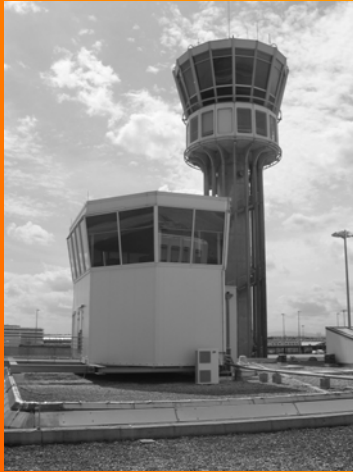
control cabin set up on a building
